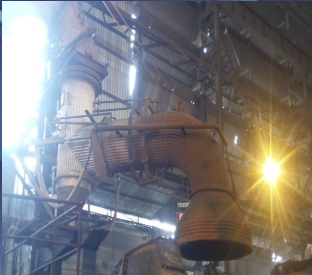
WATER COOLED HOOD & DUCT
